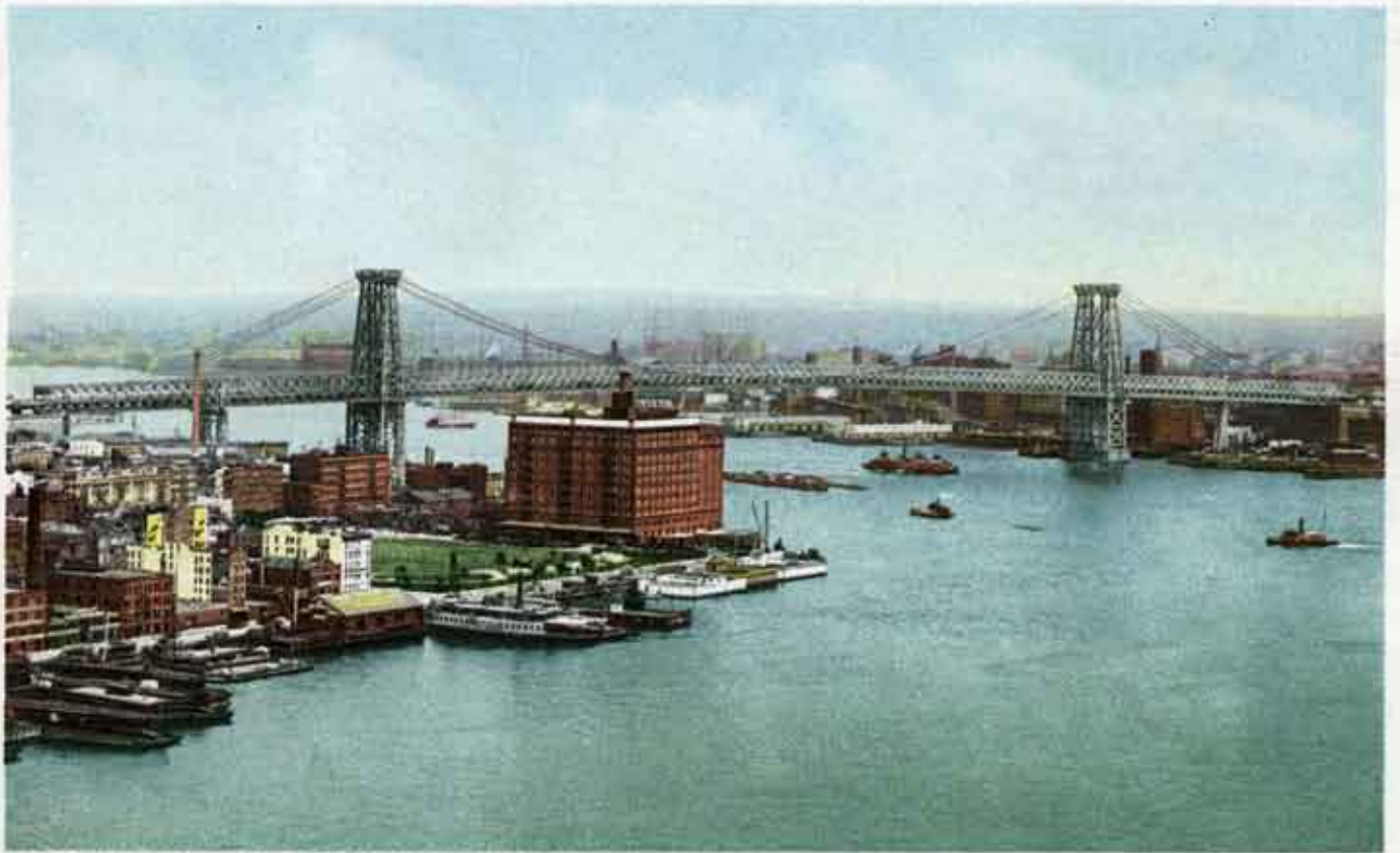
12856 WILLIAMSBURG BRIDGE, BROOKLYN, N. Y.
