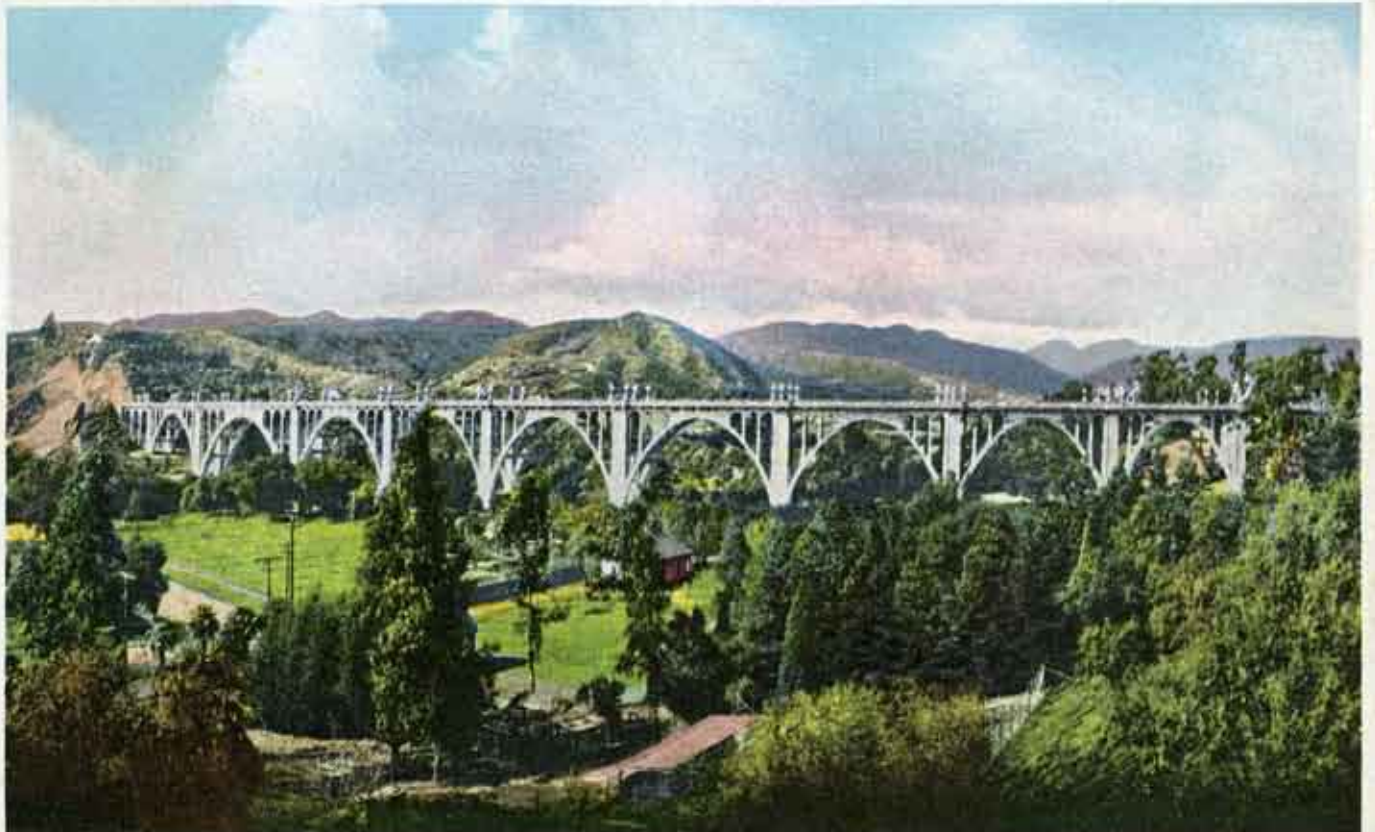
71549 COLORADO STREET BRIDGE OVER THE ARROYO SECO, PASADENA, CALIFORNIA
