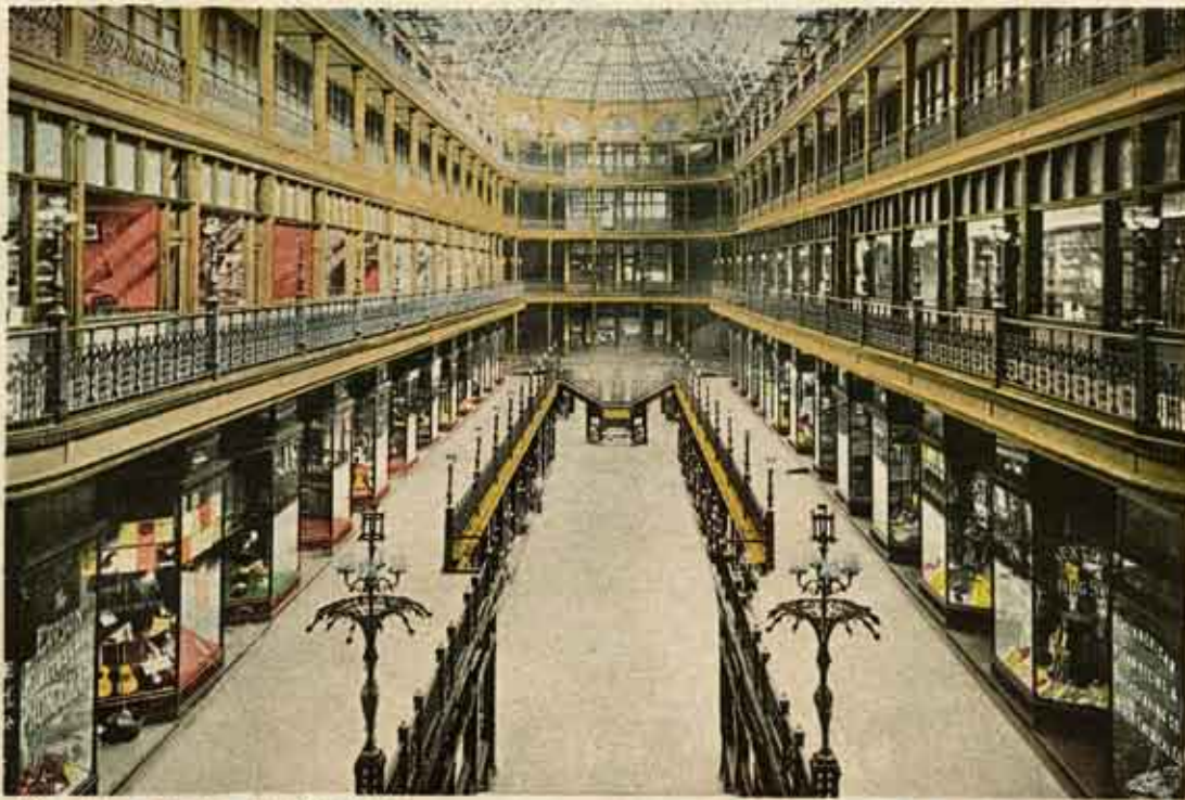
5586. THE ARCADE, CLEVELAND, O.
