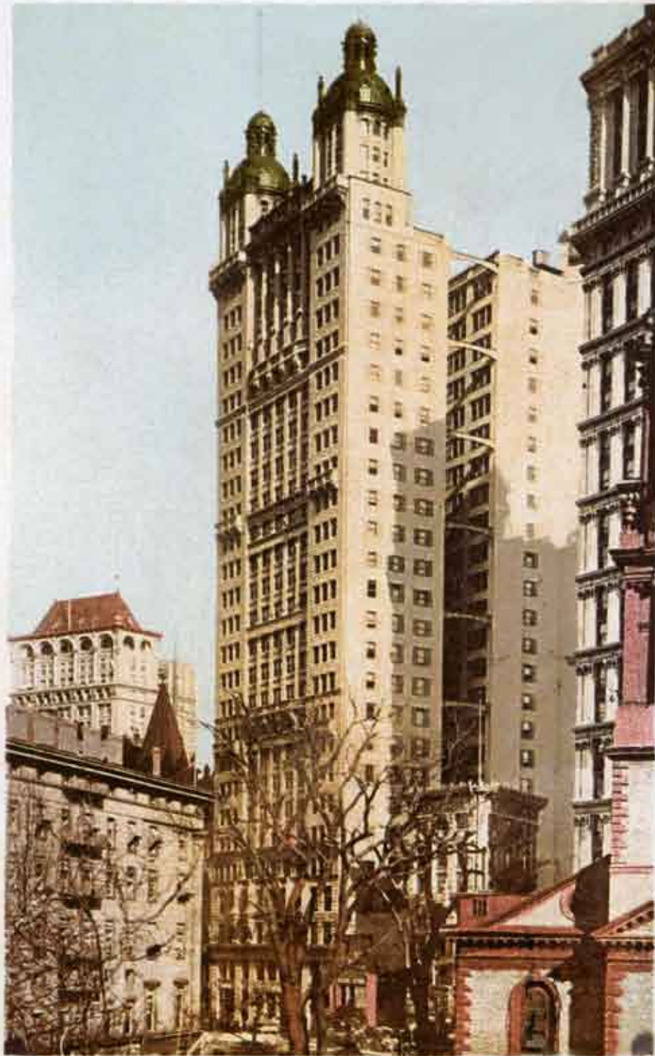
PARK ROW BUILDING, NEW YORK.
