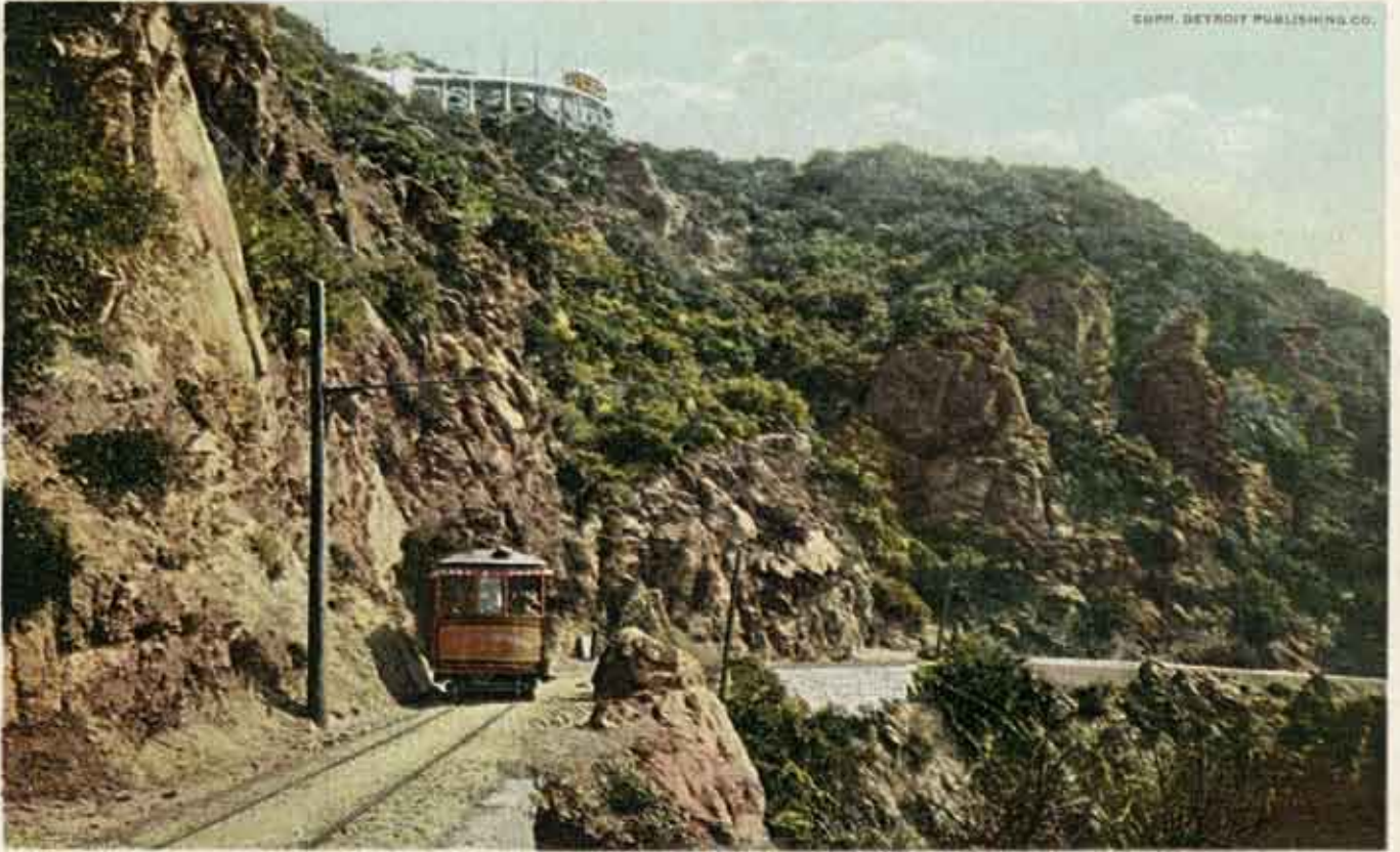
70921 TROLLEY LINE, MT. LOWE, CALIF.
