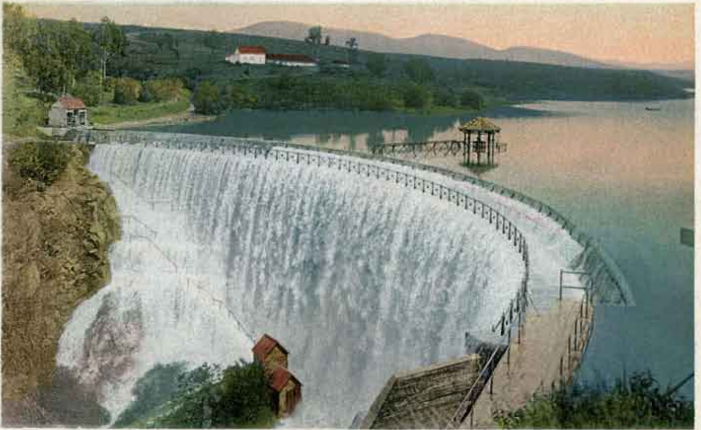
13106 THE SWEETWATER DAM, SAN DIEGO, CAL.
