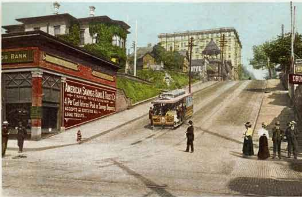
MADISON-STREET CABLE INCLINE, SEATTLE, WASH.
