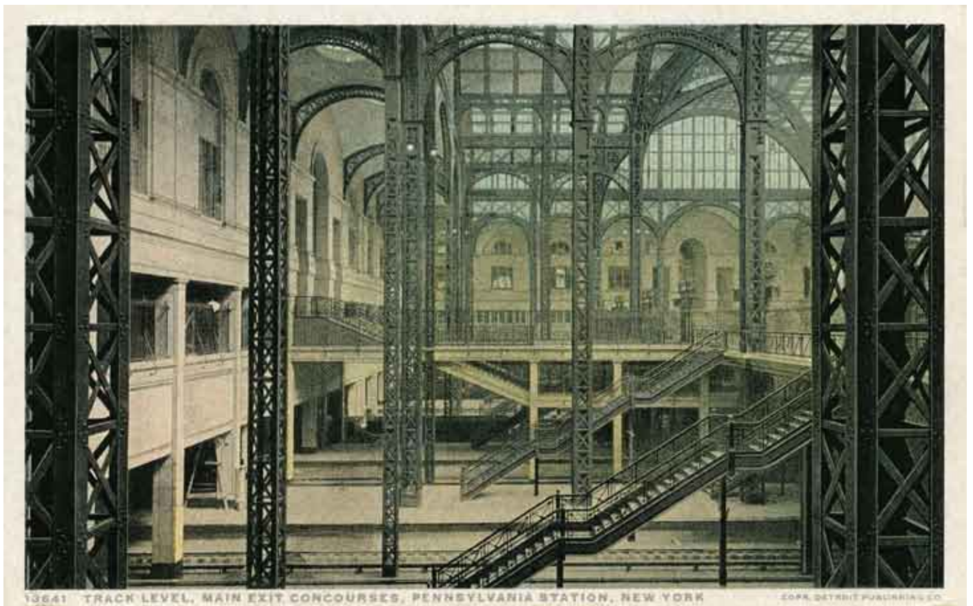
19641 TRACK LEVEL, MAIN EXIT, CONCOURSES, PENNSYLVANIA STATION, NEW YORK
